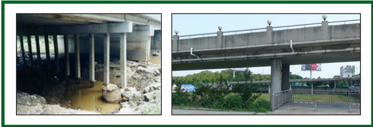
Figure 1. Wireless sensor networks placed on bridge structures
